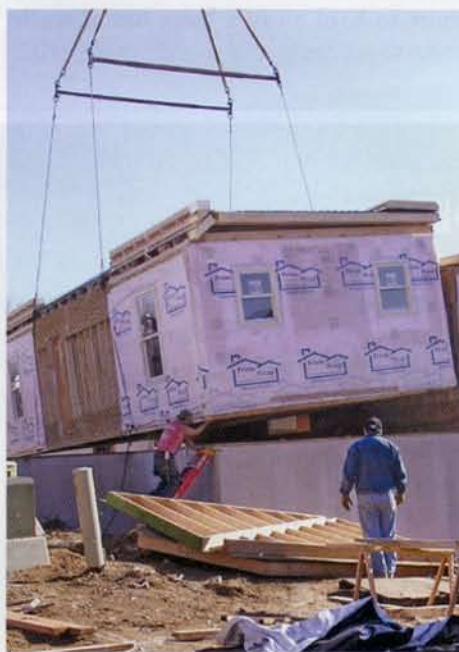
Workers guide a home onto its foundation at Hundredfold Farm.
